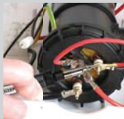
Water Heater Installation
